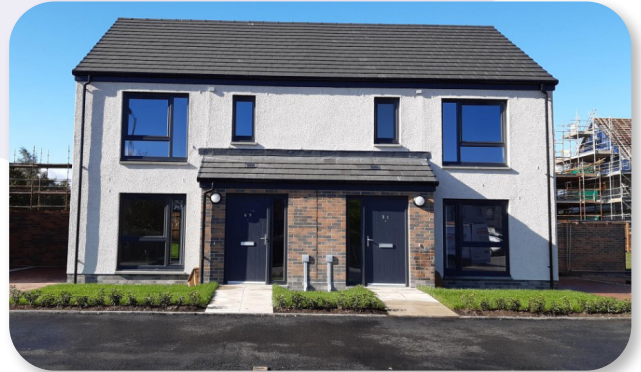
Pictured are homes from our Raploch development that will help us deliver a further 150 new build homes/2nd hand acquisitions for Stirling Council tenants in 2021/22.
